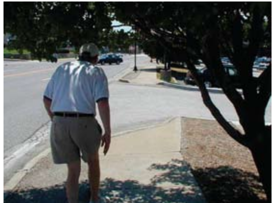
Tree branches that protrude into the sidewalk corridor must be cut or trimmed.
