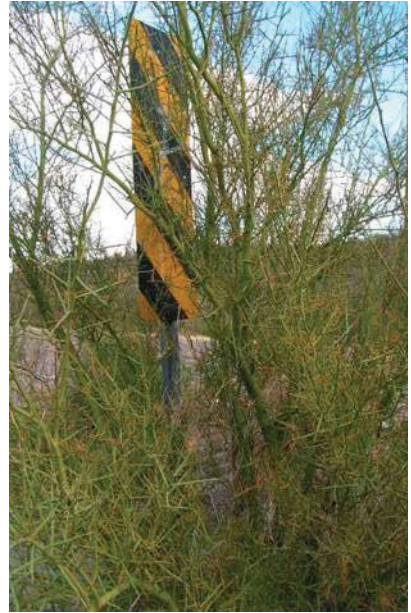
This object marker and culvert headwall are almost completely obscured by dense vegetation.
