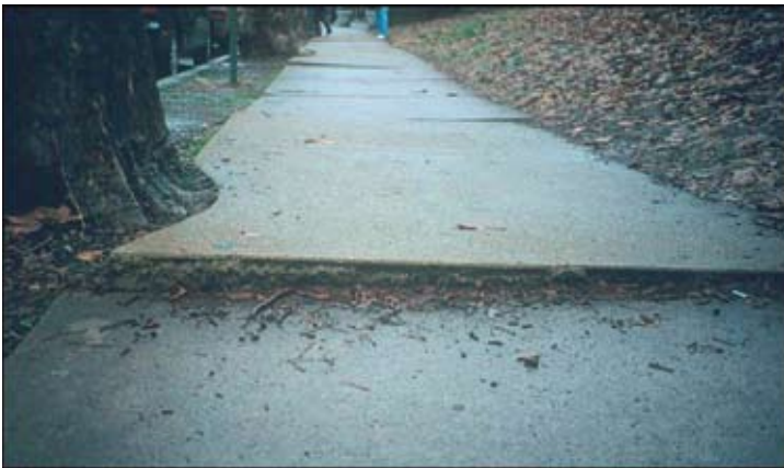
This change in level in the sidewalk due to tree roots creates a pedestrian tripping hazard and makes the sidewalk inaccessible to wheelchair users.
