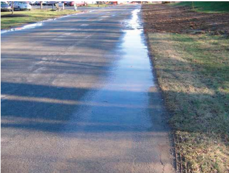
High shoulder due to vegetation growth on the shoulder prevents water from running off of the pavement, saturating the road base and causing safety problems such as ponded water (and ice in the winter).
