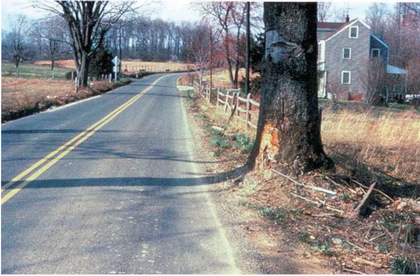
Trees near the road that have been struck before deserve special attention.
